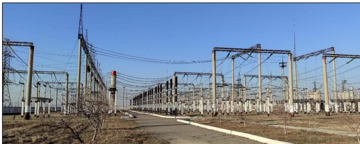
Figure 4: Substation "Tashkent" 220 kV outdoor switchgear
