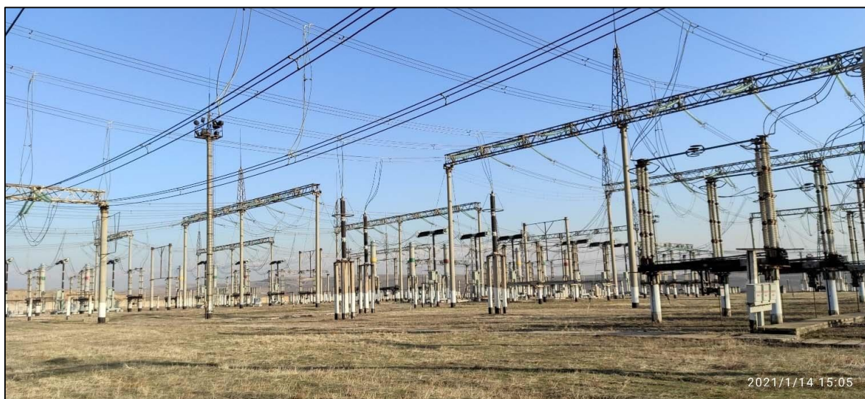
Figure 3: Substation "Tashkent" 500 kV outdoor switchgear
