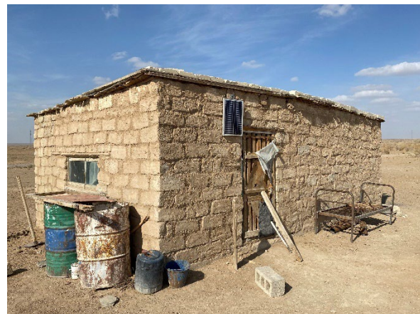
Figure 9: Buildings used by herders
