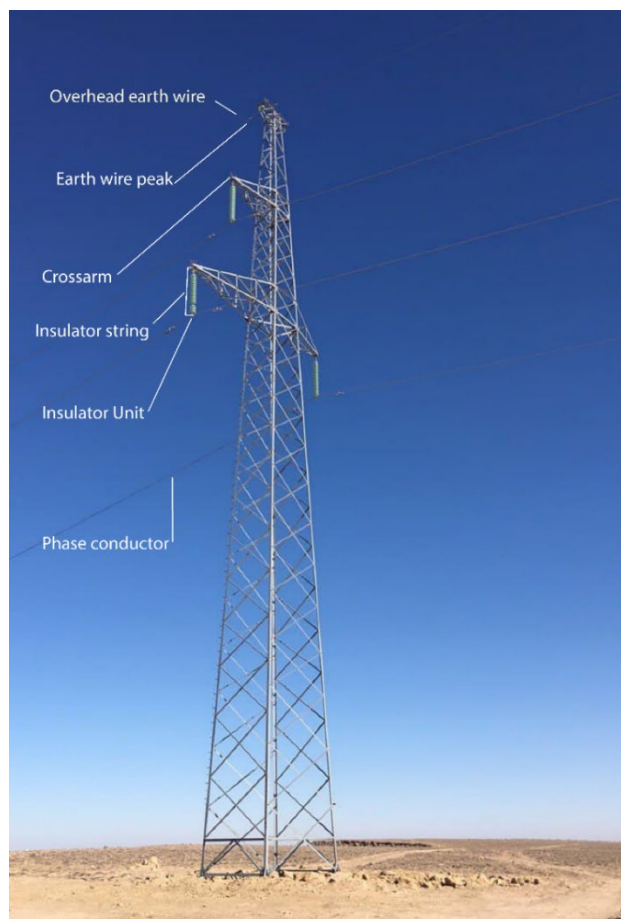
Figure 13: Components of an OHTL (source: Juru)
