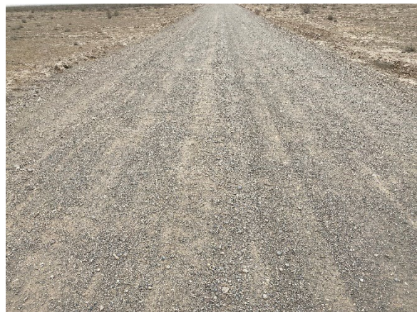
Figure 12: Access Road (from 205 km to 229 km Muruntau SS)
